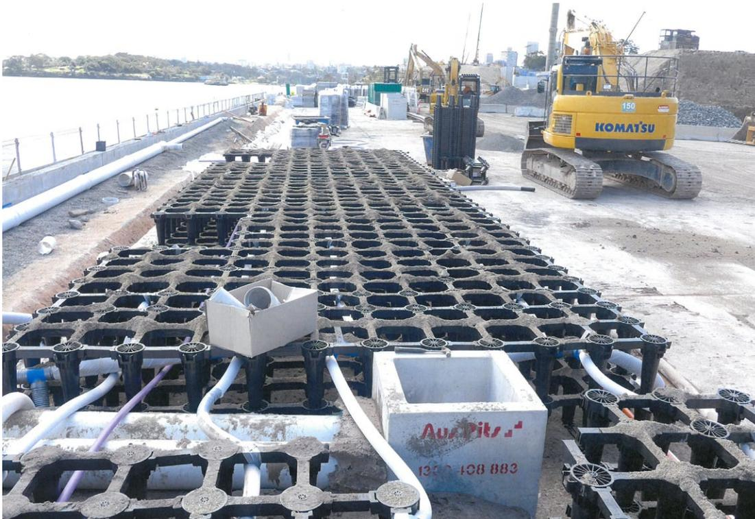
Figure 4.9 – Numerous methods are now available of integrating trees and the necessary soil volumes within urban environments while still allowing pavements and roads to continue successfully above. The above illustrates the proprietary system Strata Vault by Citygreen being used at Barangaroo Sydney.
